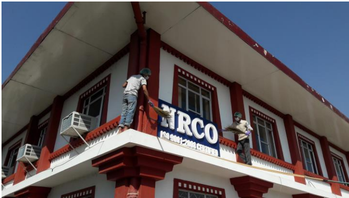
Pic: Cleaning of NRCO building,06.03.2017
